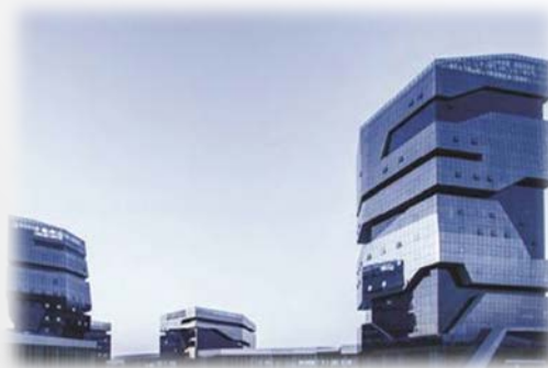
Brand-New High Tech Cashmere Industrial Park
